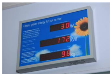
Solar Panels installed!
